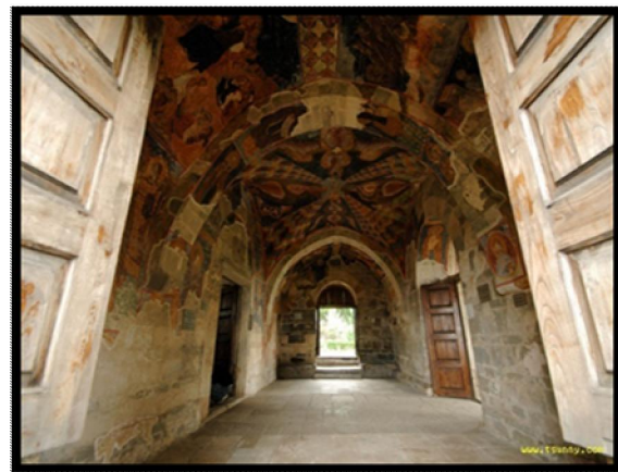
Figure 9. Inside (Entrance to the guard rooms) (gencyolcu.com)
