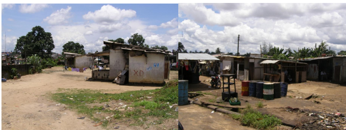
Fig.2 (c): Second Housing Types of Rainbow Town (d): Shanties within the erstwhile Rainbow Town
