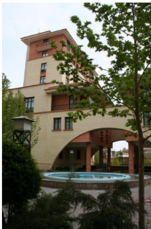
Fig. 5. View of the yard of Zeytoon Residential Complex
