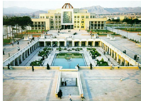
Figure 7: central courtyard of Khavaran Cultural Center with a view angle less than 9 degrees
