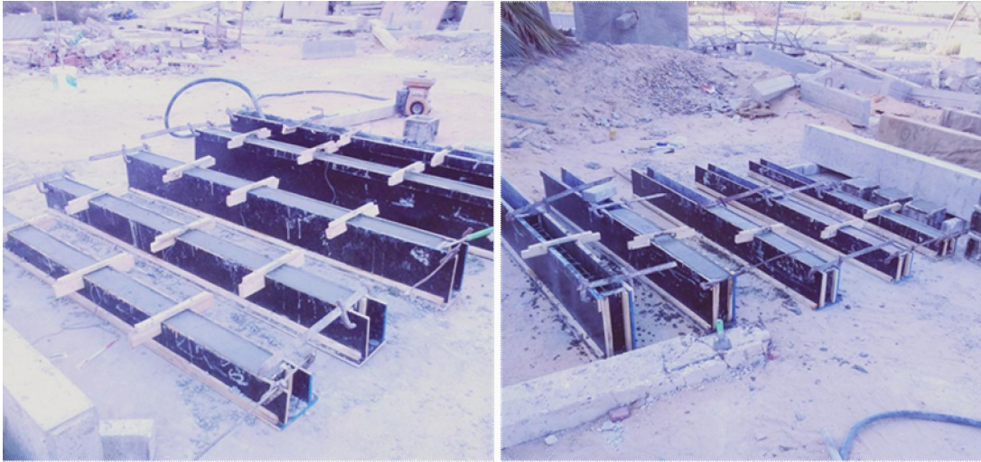
Figure [3] Wooden forms for casting
