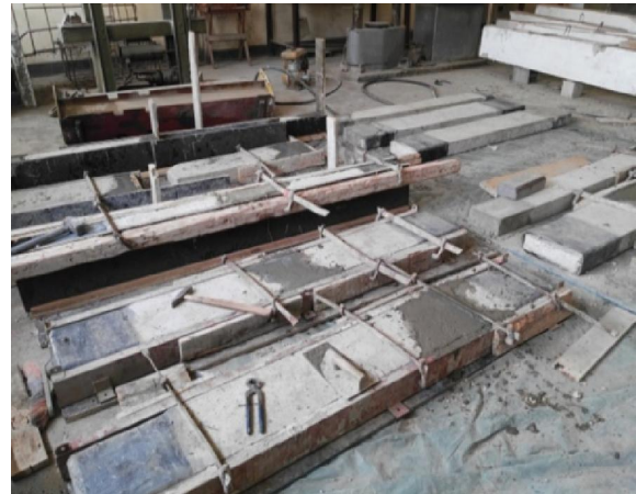
Figure [5] Replacement of damaged RC concrete by grout mortar
