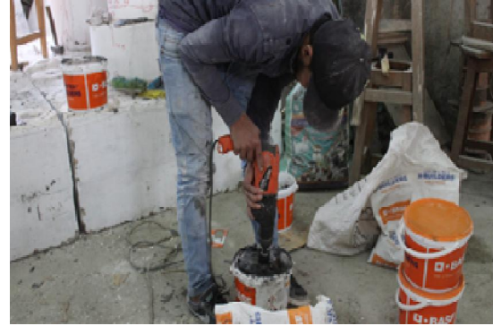
Fig. (9): Mix components using mixer
