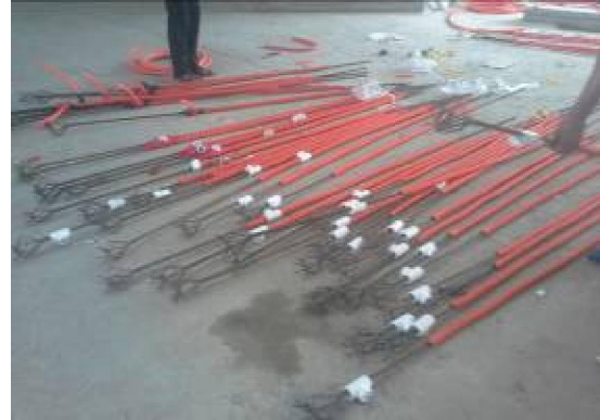
Fig. (5): Bonded Tendon with Onion End.
