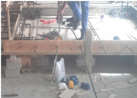
Fig. (4): Unbonded Tendon with Polypropylene Duct.
