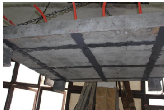
Fig. (11): Attachment of CFRP strips
