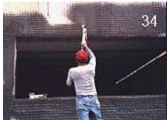
Figure 2: EPS system plastering works using shotcrete
