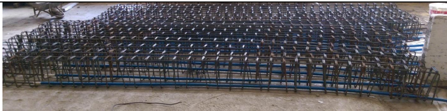
Fig (4) Reinforcement cages
