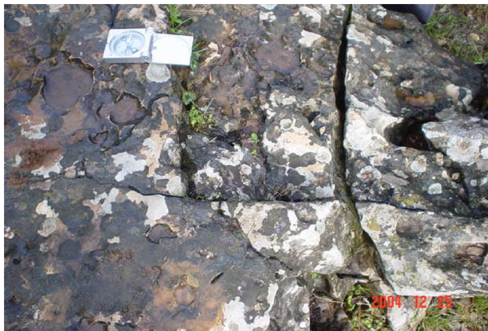
Figure 2. Limestone rock shows fractures and joints at the surface over the cave area.
