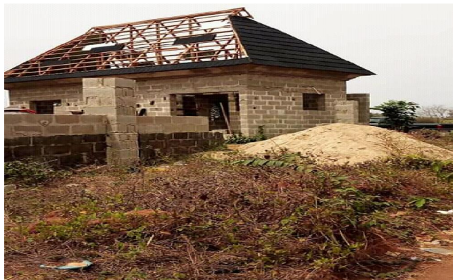
Plate 3: Ongoing roof truss construction of a duplex in Marine Base and bungalow in Igwuruta
