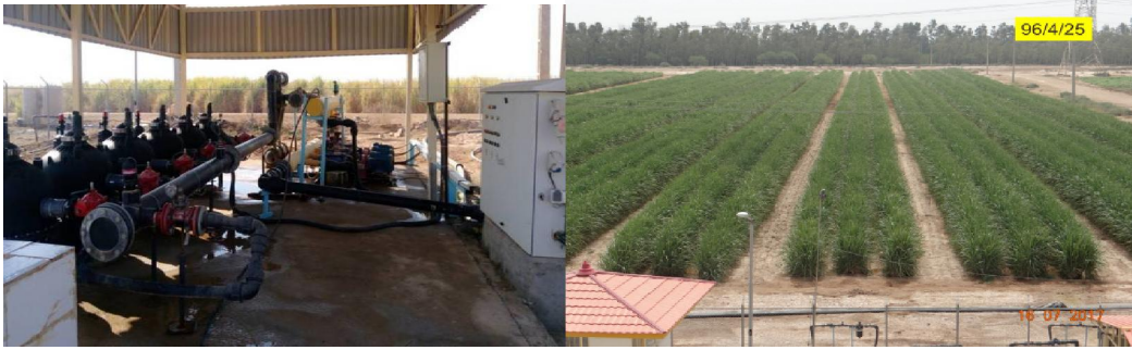
Figure 5. Pumping and filtration station and observation the subsurface drip irrigation farm
