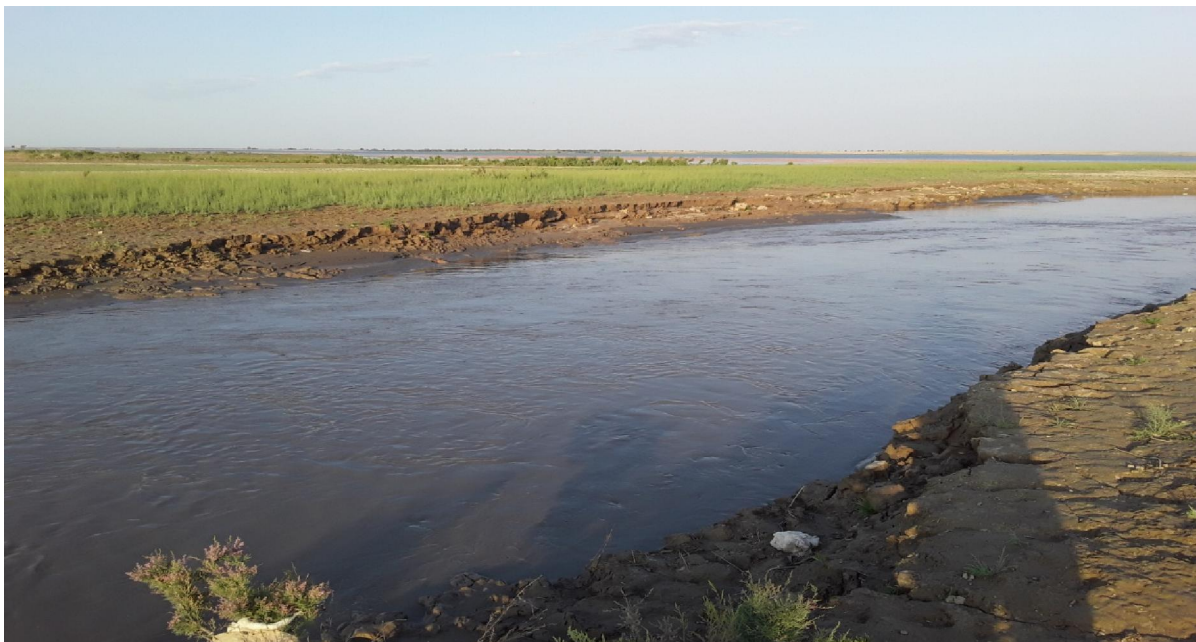
Photo 1. Location of the Tuatortar Canal to the Jizzakh Reservoir
