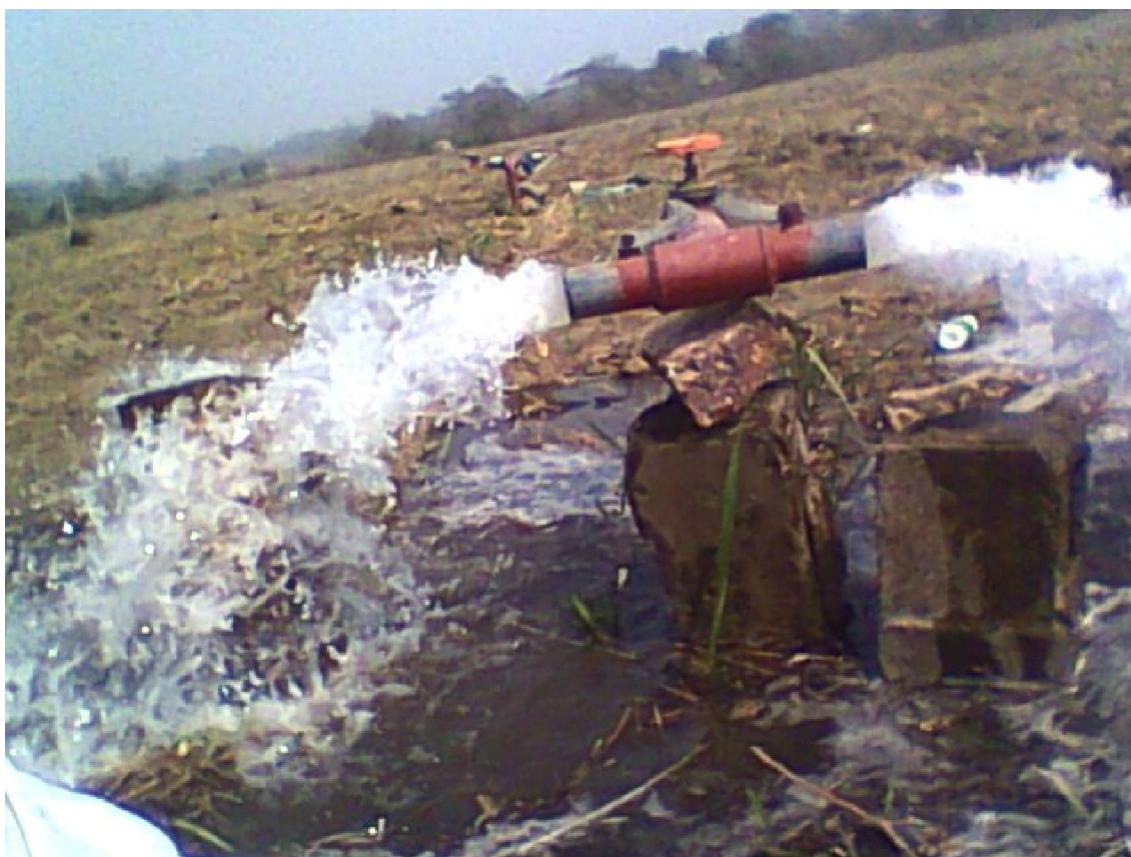
Central pump system, before hoses were inserted, at an irrigation scheme in the LNRBDA
